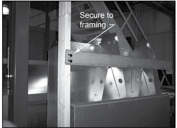
Figure 12.14 Secure to Framing
